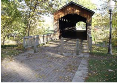
Ada Covered Bridge
