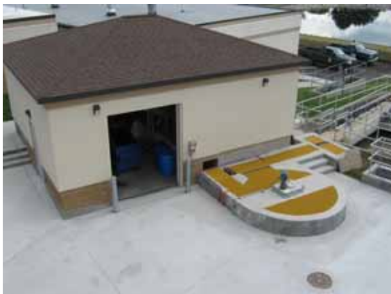
New headworks building
