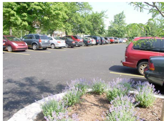
North Parking Lot Porous Pavement
