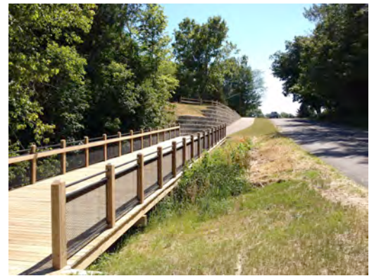
Retaining Wall & Boardwalk along Greenly Street
