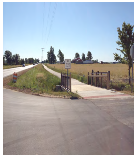
HMA trail and boardwalk along Byron Road
