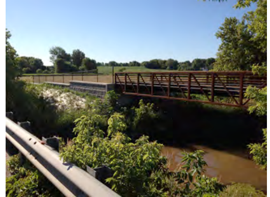
Non-motorized Trail Bridge and North approach
