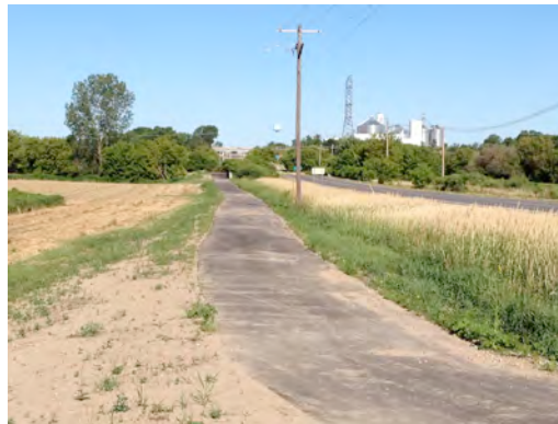
Trail approaching prefab bridge along Byron Road, Zeeland Township
