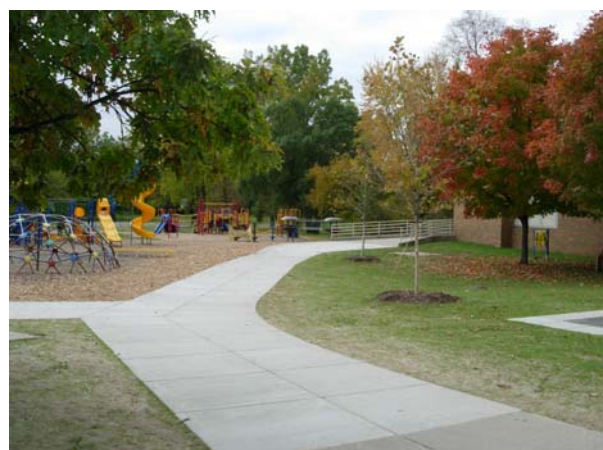
Playground Drainage Improvements
