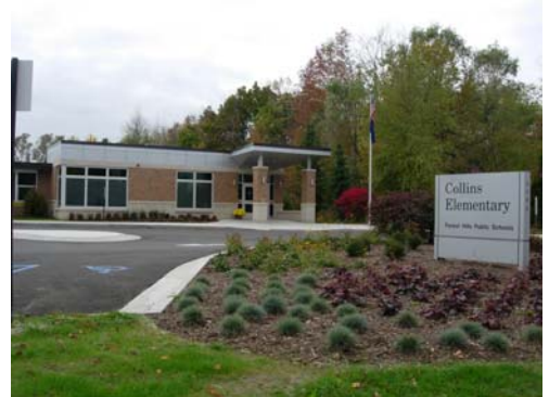
New Front Entrance
