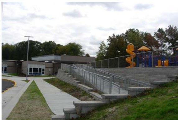
Playground access ramp
