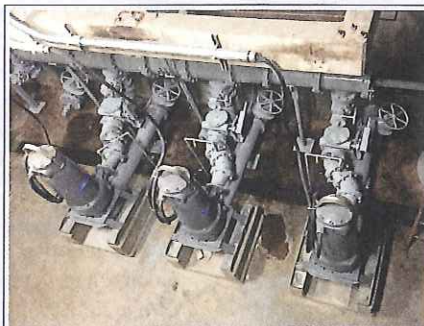
Closed loop cooling of the motors eliminated seal water piping, seal pots and the compressor.
