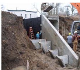
Thanksgiving Afternoon Install Wingwalls
