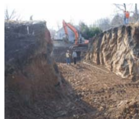
Wednesday Afternoon Excavation Complete
