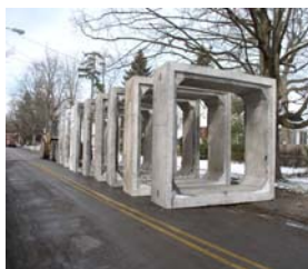
Precast Tunnel Sections
