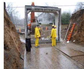
Thanksgiving Morning Place Precast Sections
