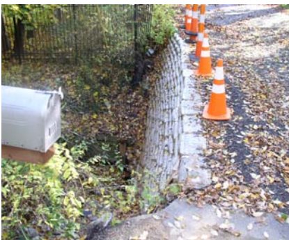
Temporary Headwall Shoring after Pre-Project Washout
