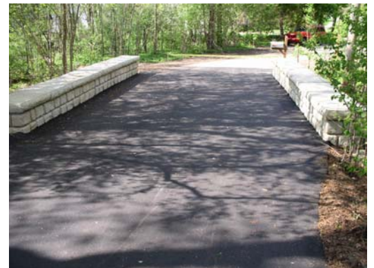
Final Residential Drive over New Culvert
