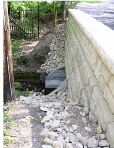
Modular Block Headwall over Box Culvert
